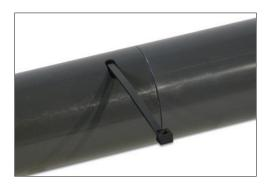
Figure 5-4 Push Shear Tie Through the Window
