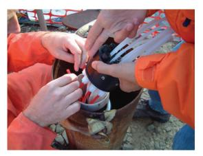
Figure 9-3 Pump Tubing Being Attached to a Wellhead
