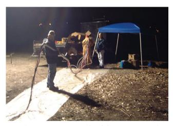
Figure 4-5 Casing Section Being Threaded Over Monitoring Tubing
