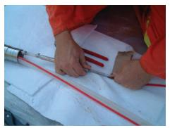
Figure 6-11 Using Sand Paper to Push Tubing onto Pump Stem
